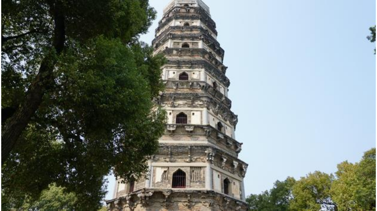
PHOTO: This leaning Cloud Rock Pagoda is a 7-story, the 10th-century octagonal pagoda built entirely of brick. (Photo by Chelsea Davis)
